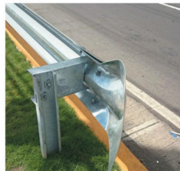
◎C立柱连接图/C Post Connection Diagram
